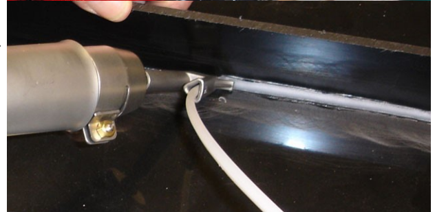
Welding using Speed nozzle
